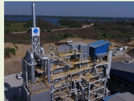
WtE plant completed in April 2017 in Yangon
